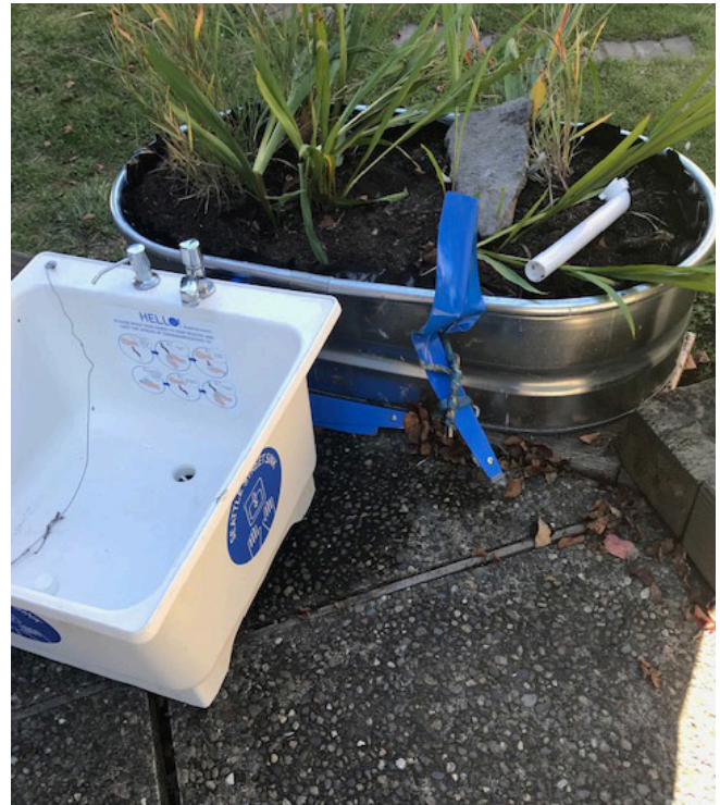
Figure 7. Sink damage from vandalism. Aaron Allen.
